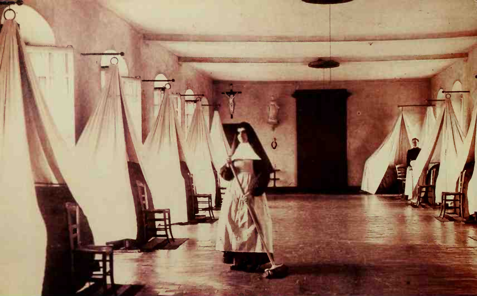
The school dormitory
